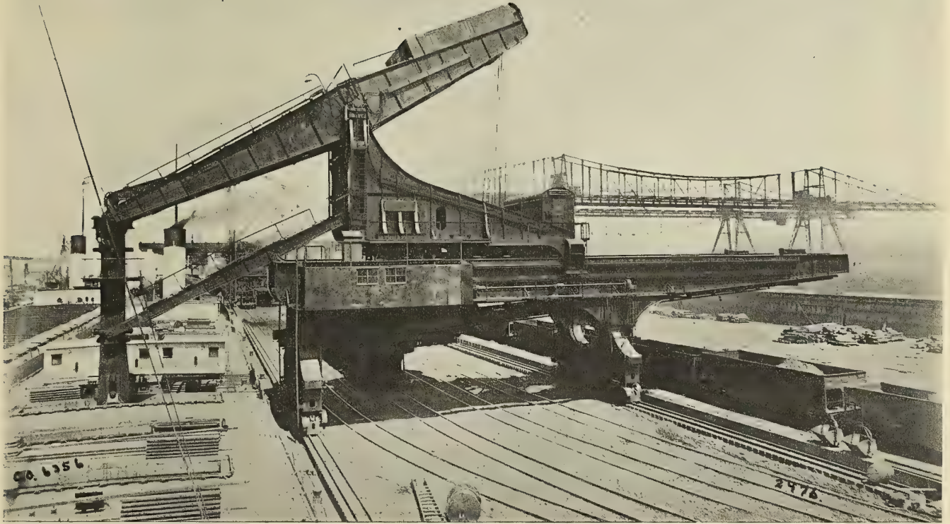
Fig. 2.—Wellman-Seaver-Morgan Unloader Installed at the Docks of the United States Steel Corporation, Conneaut, Ohio. There Are Seven of These Unloaders Installed at This Plant, Some of Which Are Shown in the View Above
